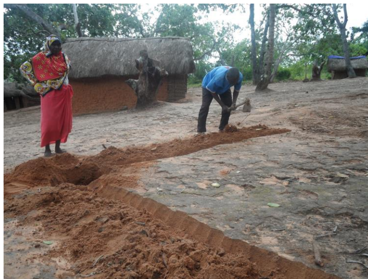
Figure 6: V-shaped micro-catchment
